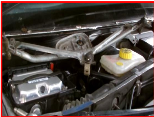
Wiper linkage susceptible to rust and other contamination.
