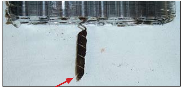
Image 4 The image reveals how foreign matter collects on the turbulators, which accelerates the corrosion process of the U-bends.
